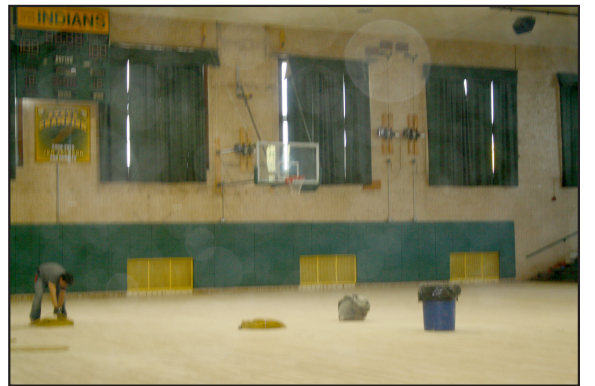
A worker refinishes the new floor in Gym One.
